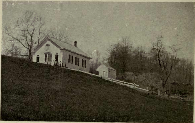
A hillside schoolhouse
